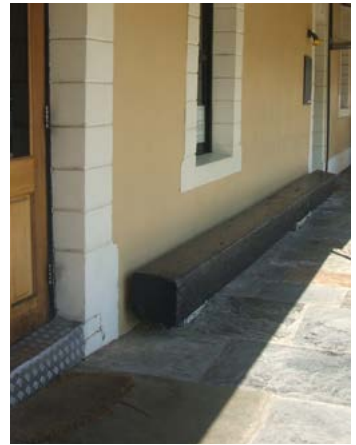
Sawn pile on the verandah of the Williamstown Hotel, 2020 (Image courtesy of the author).
